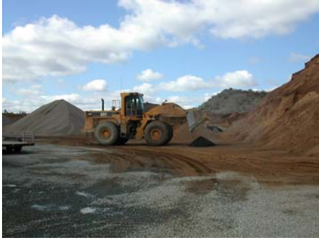
c. Aggregates in an asphalt plant in Michigan
