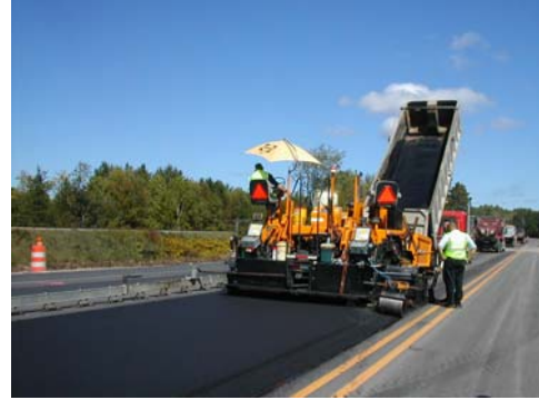
d. Asphalt concrete construction in Michigan
