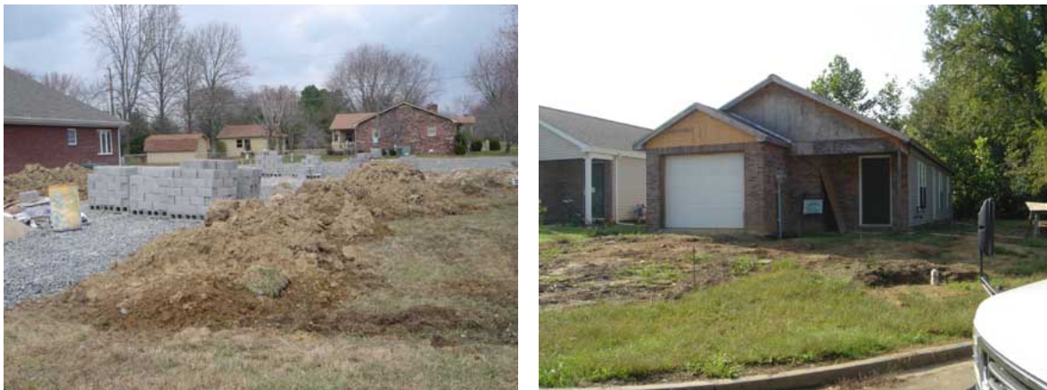
Fig. 2: Habitat Houses During Construction
