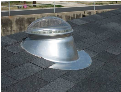
Figure 1: Skylight Installation
