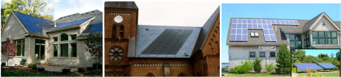
Figure 8: Patchwork Placement of Solar Collection Panels
