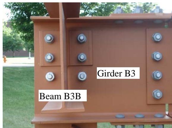
Figure 1 – View C Double bolted-welded-angle shear connection, back of View B
