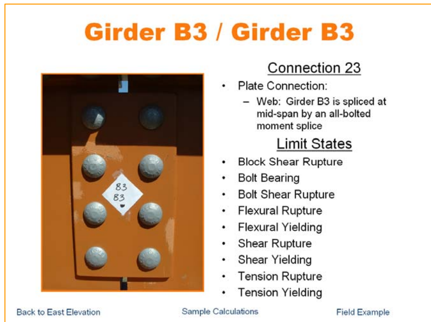
Figure 5 Close-up view of connection 23 and the list of limit states this connection should be designed for.
