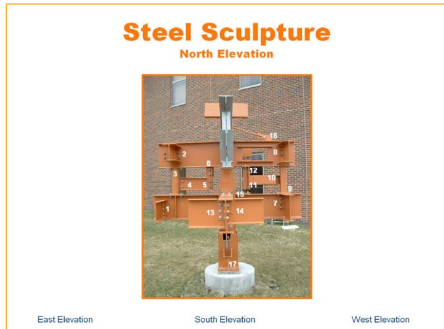
Figure 3 North Elevation view of steel connection sculpture.
