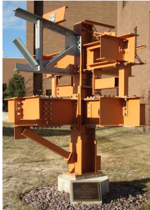
Figure 2 8-ft tall steel connection sculpture at Minnesota State University
