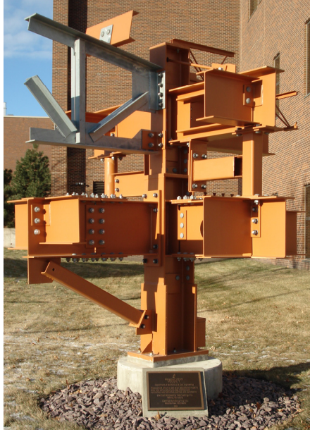
Figure 2. The 8-ft tall steel connection sculpture at Minnesota State University
